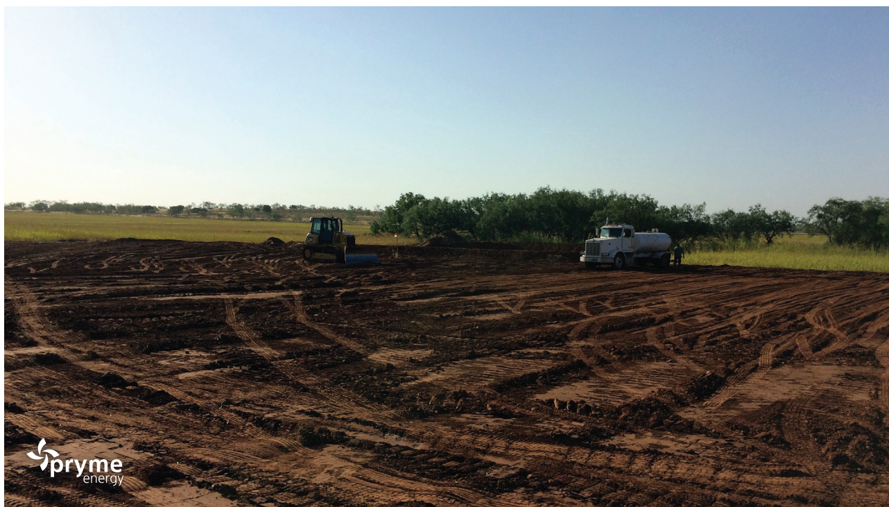
Site preparation on the Hopes-Boles PU #1 well
