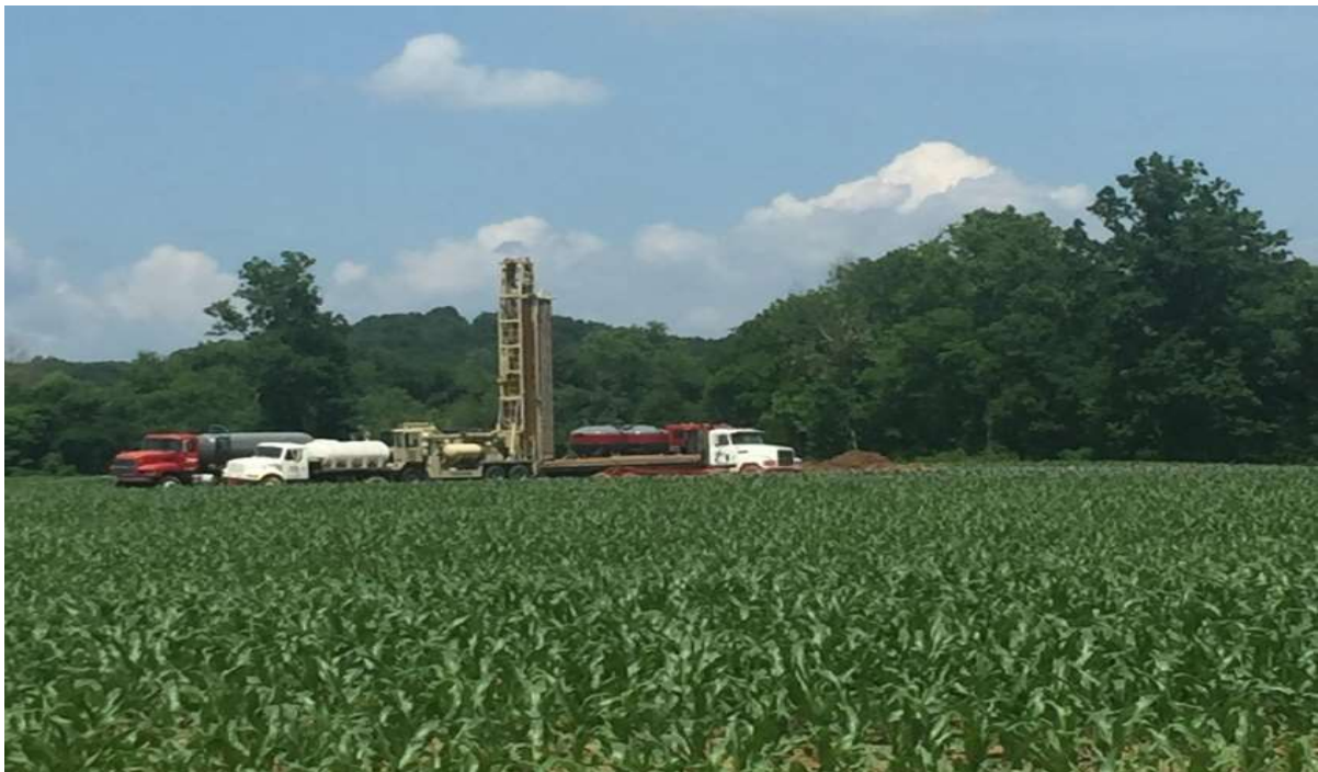
Figure 3 – Drilling the Weldon-Young #1A well in Kentucky.
