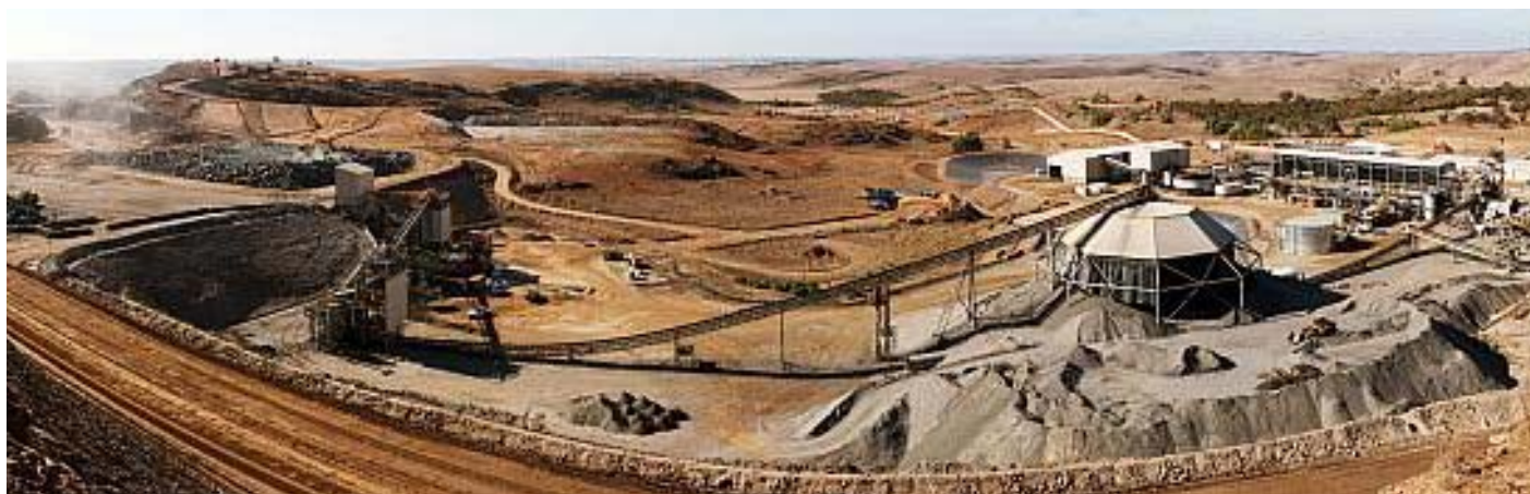
Left: ROM pads and crusher facility. Right Foreground: Crushed ore stockpile, adjacent to and under the dust containment cone
