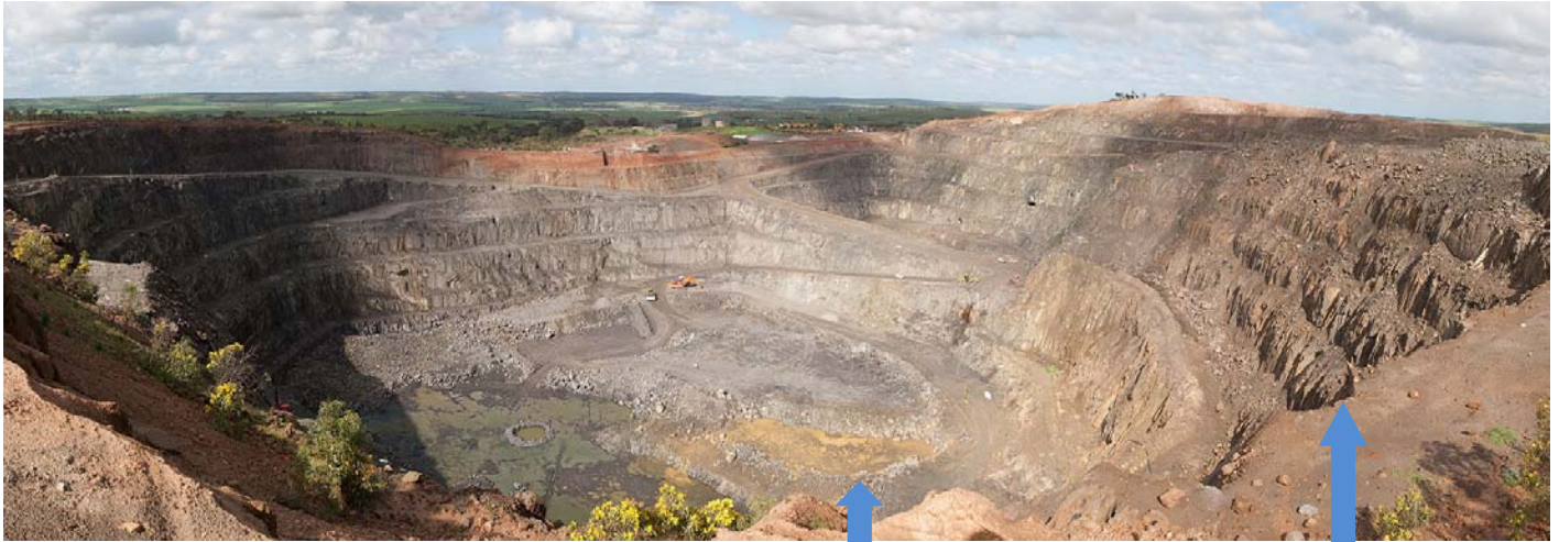
Photo: View of Kavanagh Pit showing base of old Kanmantoo Mine pit and the original Kanmantoo Pit wall .
