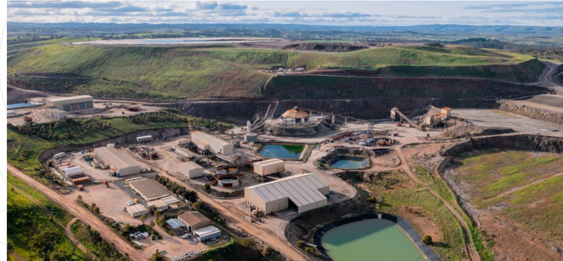
3.6MTPA PROCESSING PLANT
