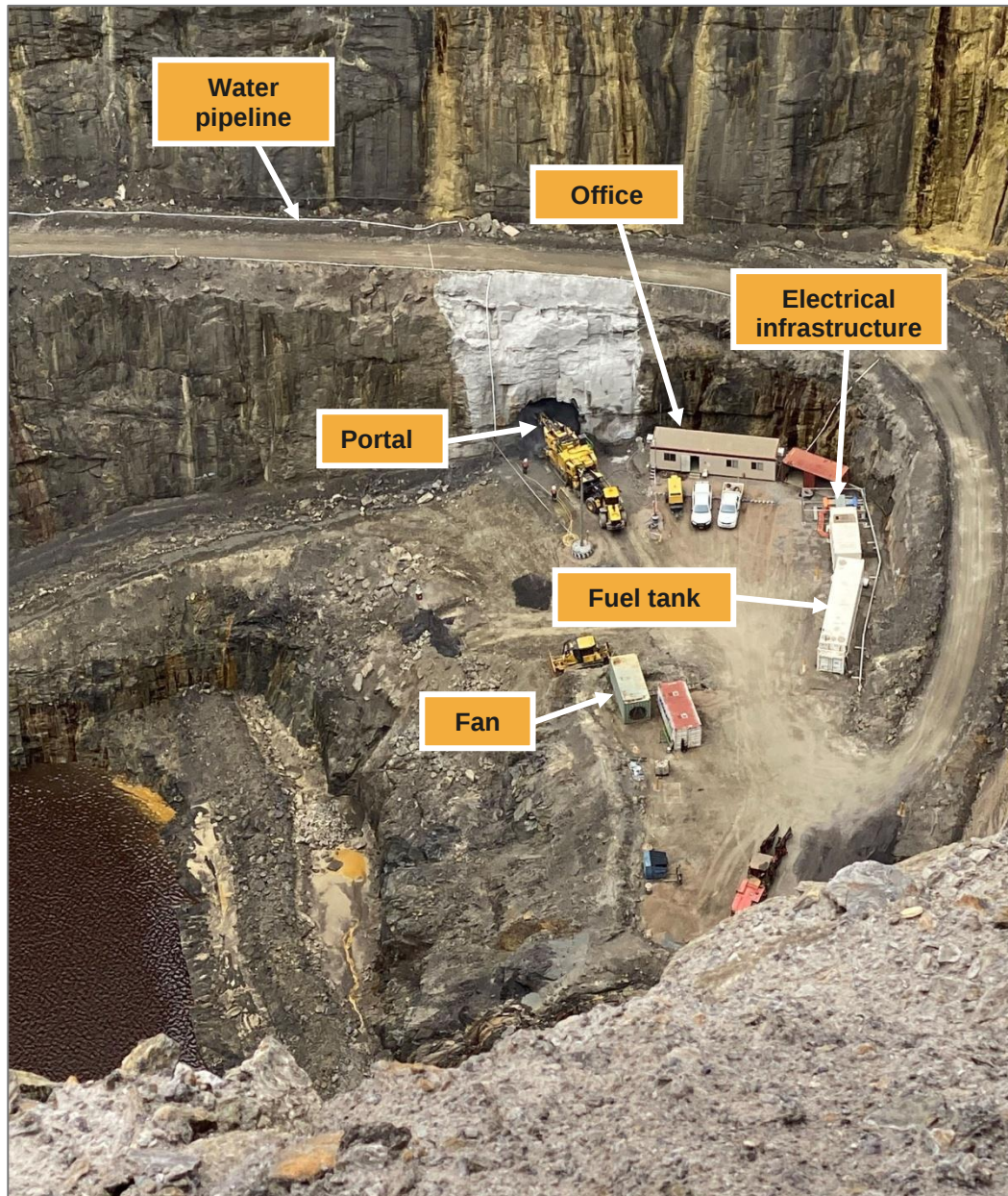
Figure 52: Infrastructure located at the underground portal
