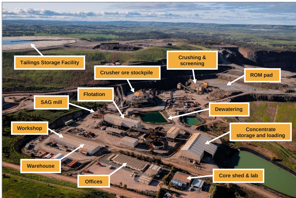
Figure 40: Kanmantoo Copper Mine processing plant and workshops
