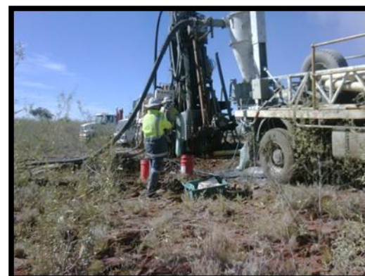
Drilling at Yanco Glen
