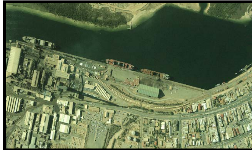
Port Pirie common berth facility
