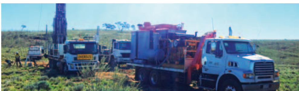
Drilling at Yanco Glen
