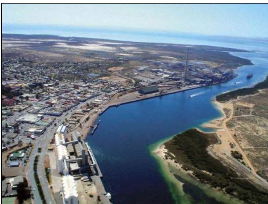
Figure 1 Aerial view of Port Pirie
