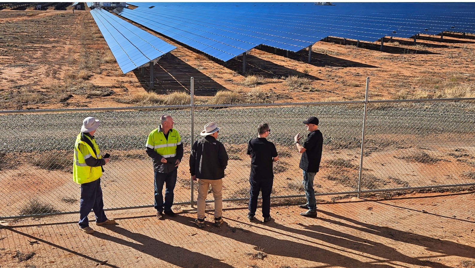
Image 6 Broken Hill 53MW Solar Farm
