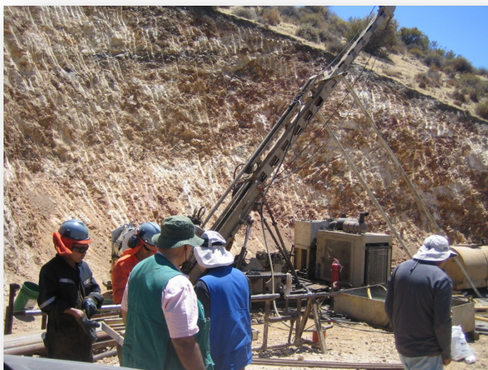
Drilling at the Joshua Project, Chile 2012
