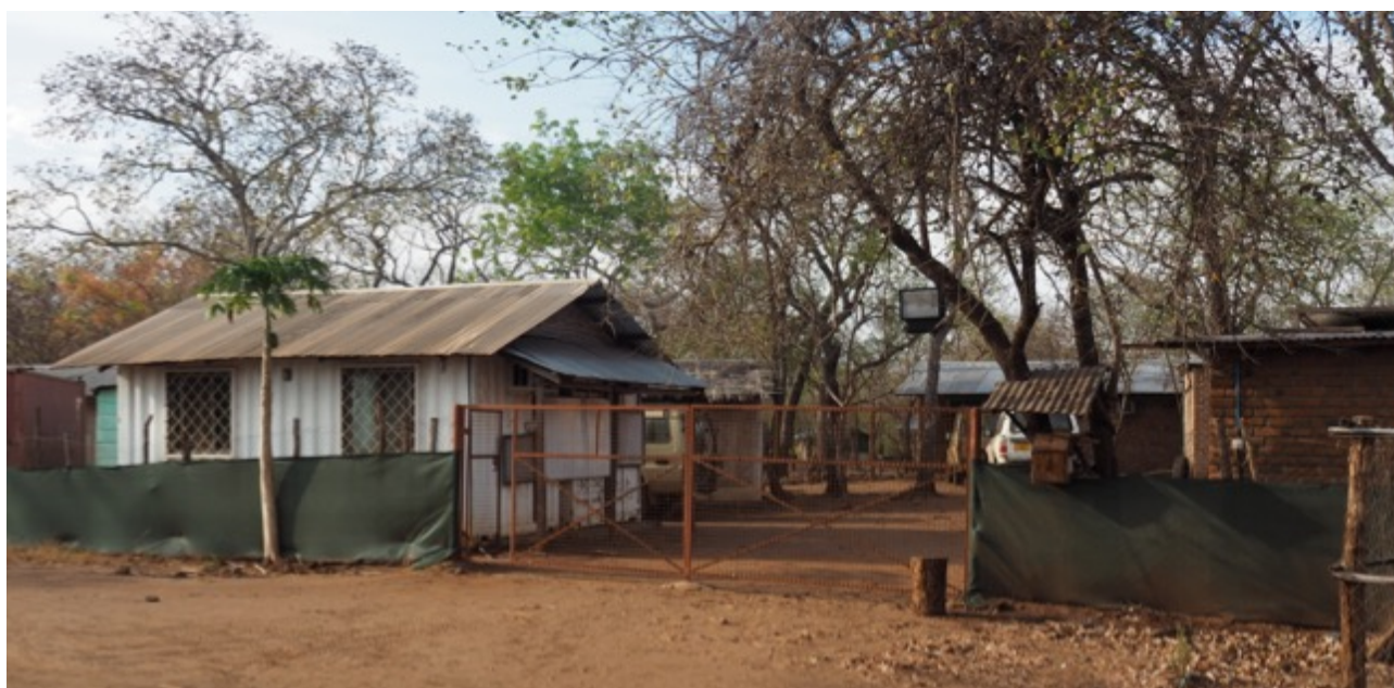
Figure 5 – Ntaka Hill camp offices
