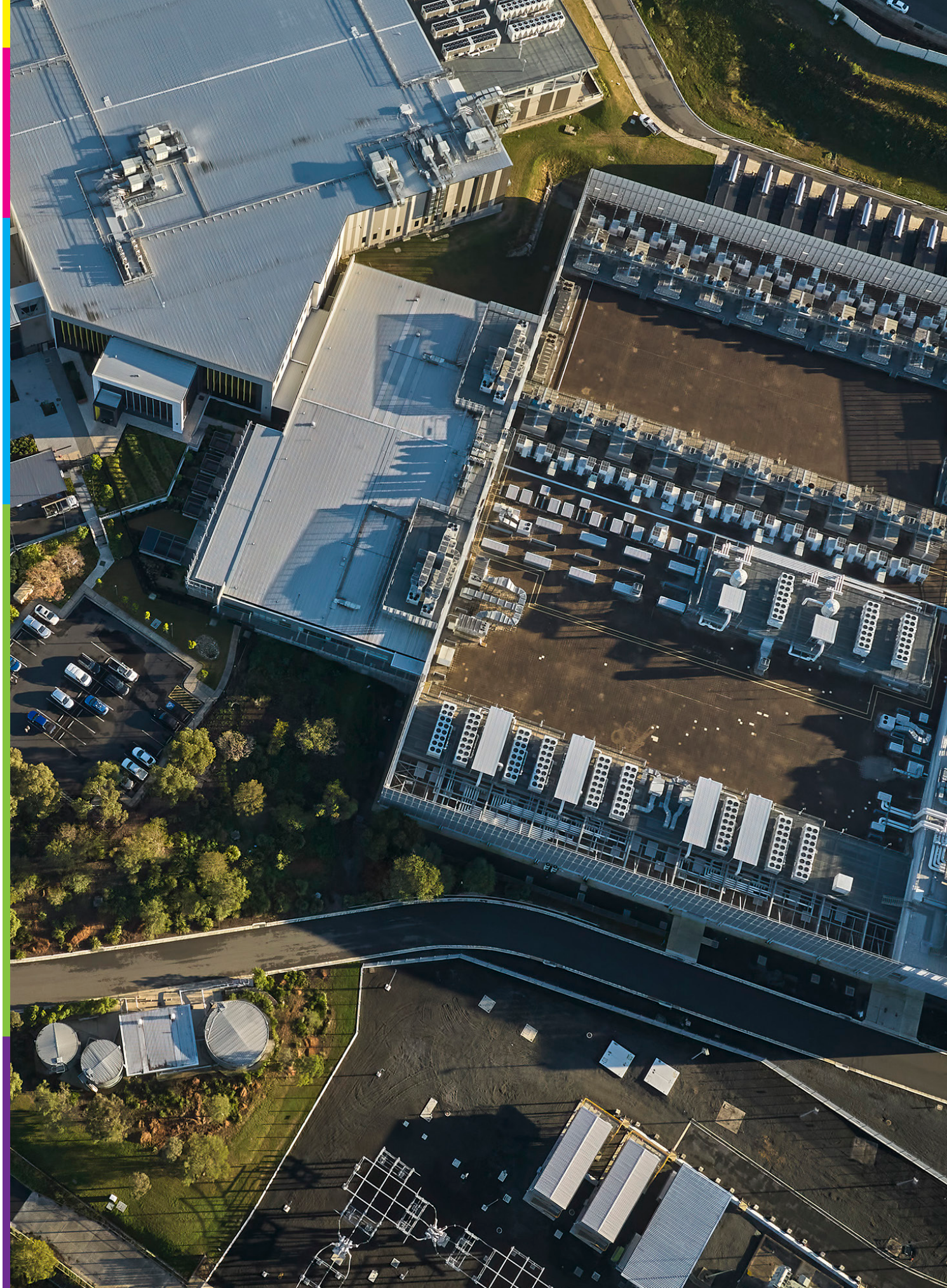
Eastern Creek data centre
