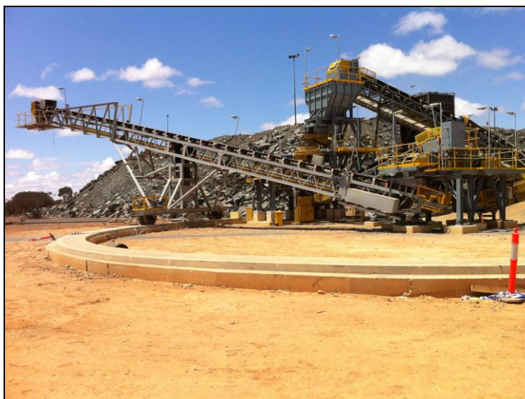
Photo: HMS Plant under construction 24 October 2011.
