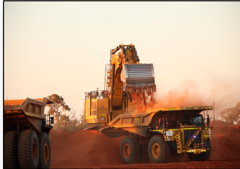
Preparation for mining
