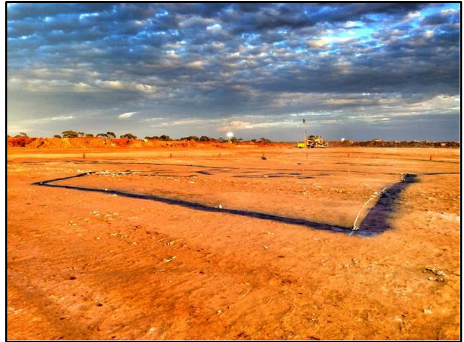
First Ore Mark Up – Havana Pit
