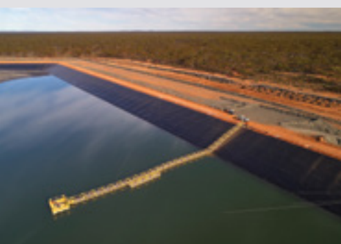
Nova Operation Tailings Storage Facility
