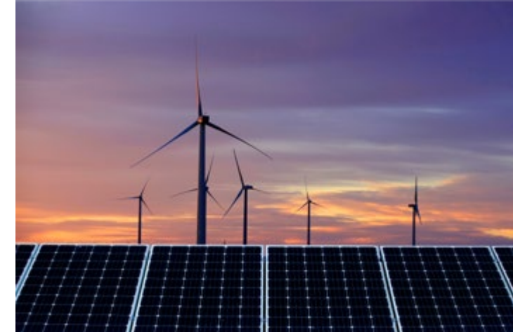
Renewable Energy Generation
