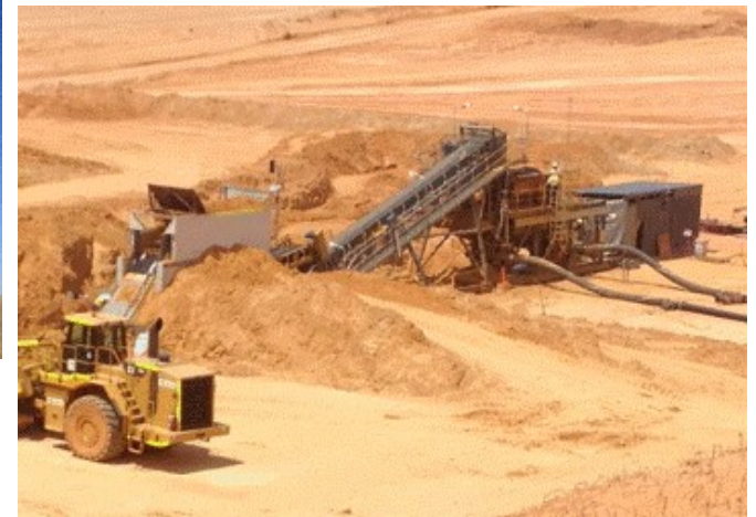
Mine Slurry Unit
