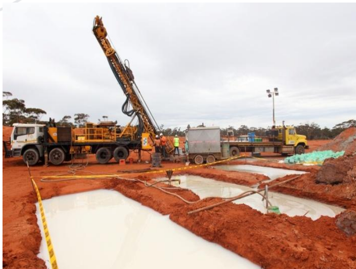
Traditional drilling fluid sumps
