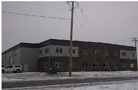
New Calgary manufacturing facility
