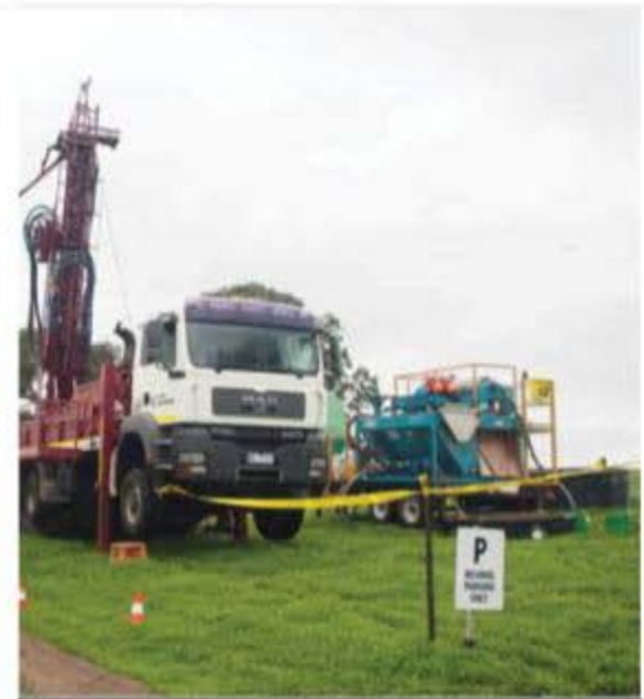
No sumps – closed loop system
