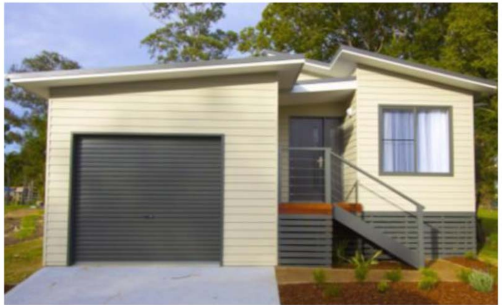
New home on-site at The Grange
