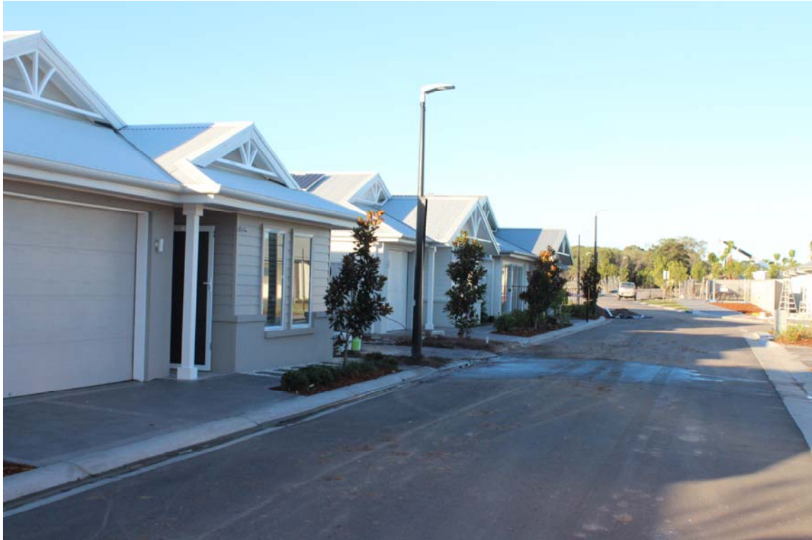
New homes now settling at Latitude One, NSW Coast.
