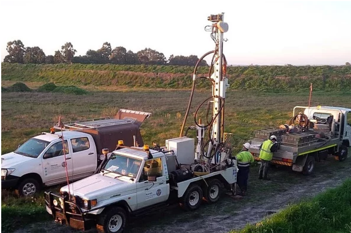
FIGURE 3 : MANTIS 75 DRILL RIG AND SUPPORT TRUCK
