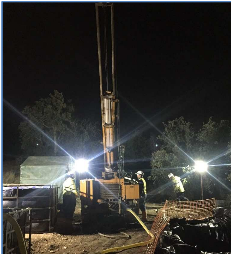
FIGURE 1: GEONOR DIAMOND DRILL RIG ON SITE AT SAN JOSE WITHIN THE AREA MARKED IN FIGURE 2.
