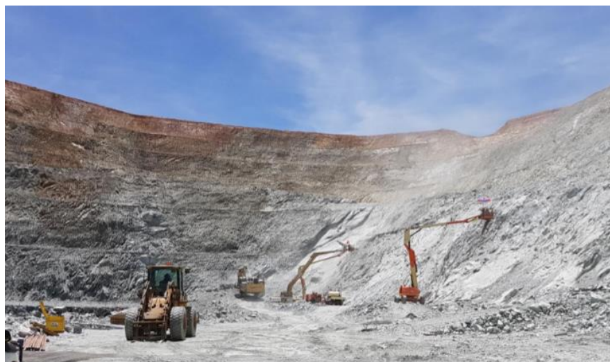
Photo 2: Cannon Open Pit Ground Support Drilling (19 November)
