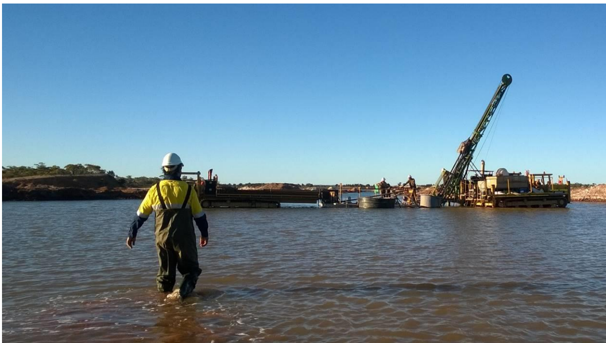
Photo 1: Drilling GLD001 at Doughnut Jimmy
