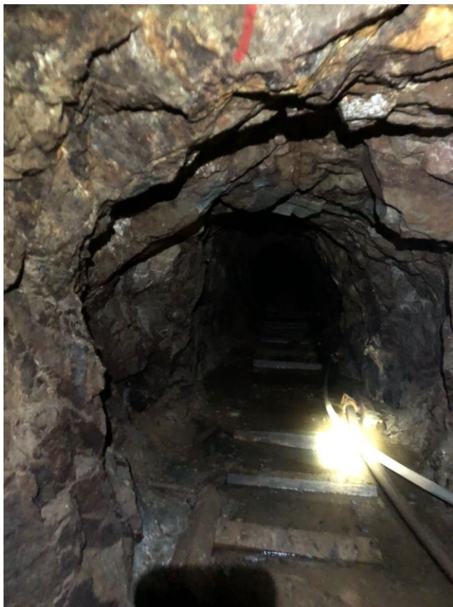
Photo 3: Old railway sleepers still in place in the floor of the main access adit.
