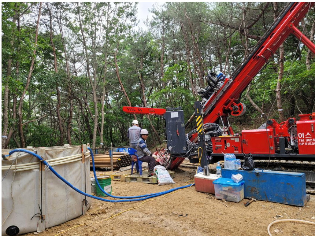
Photo 1 – Drilling at Nettle, Deokon Project
