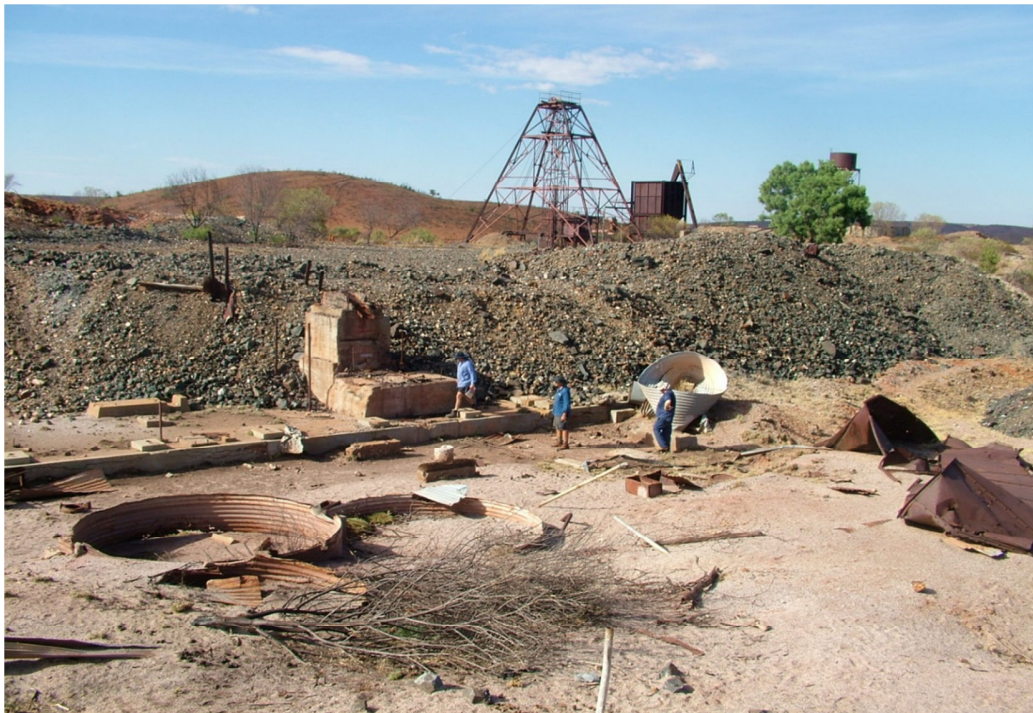
Figure 3 – Photograph of the Pioneer headframe in the background, Old Battery site and tailings in the foreground
