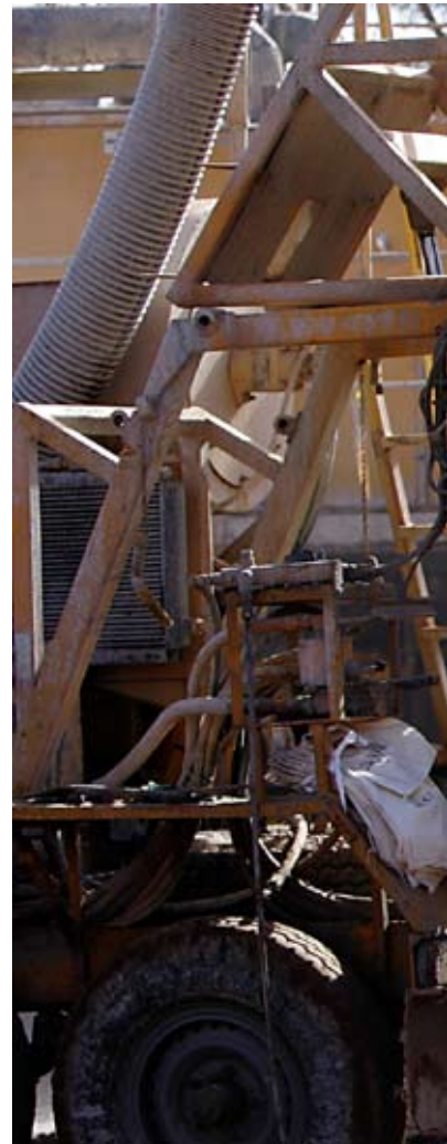
Drilling at Jungle Dam
