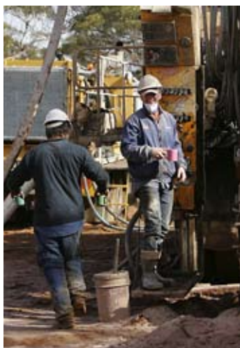
Drilling at Jungle Dam
