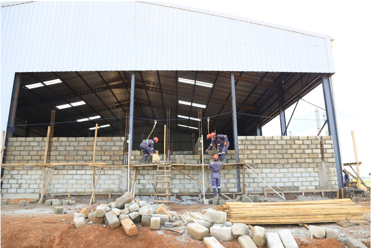
Figure 4: Construction of Technical Facility laboratory brickwork.
