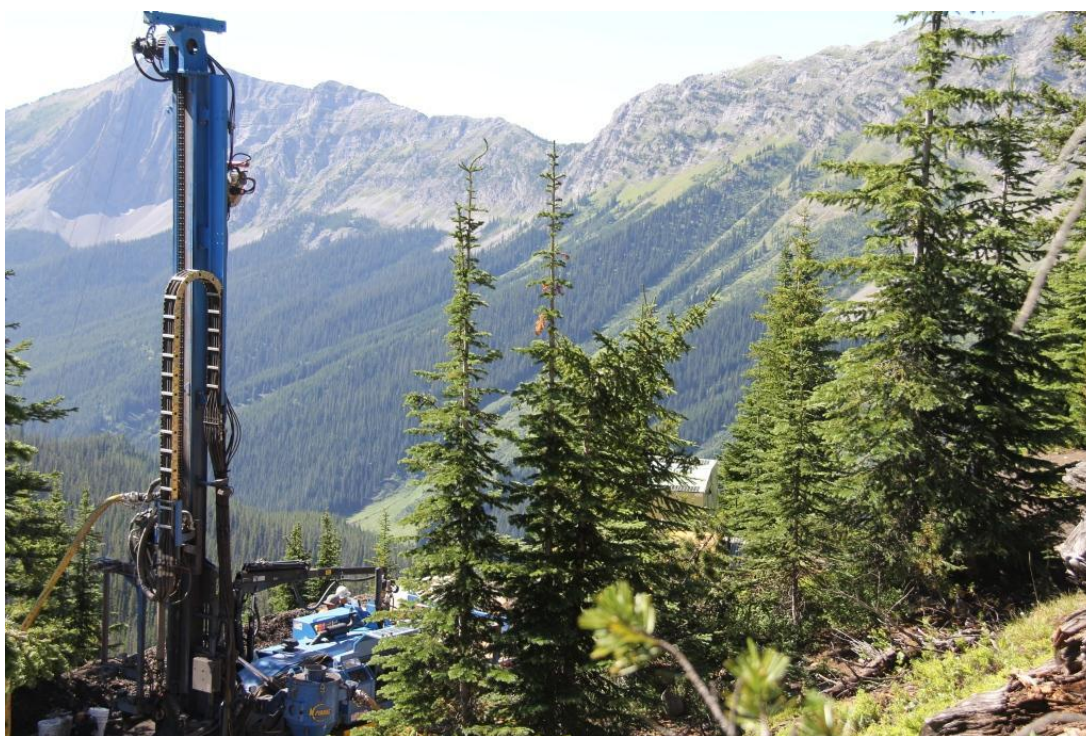
Figure 3 – Drilling Activity –Crown Mountain North
