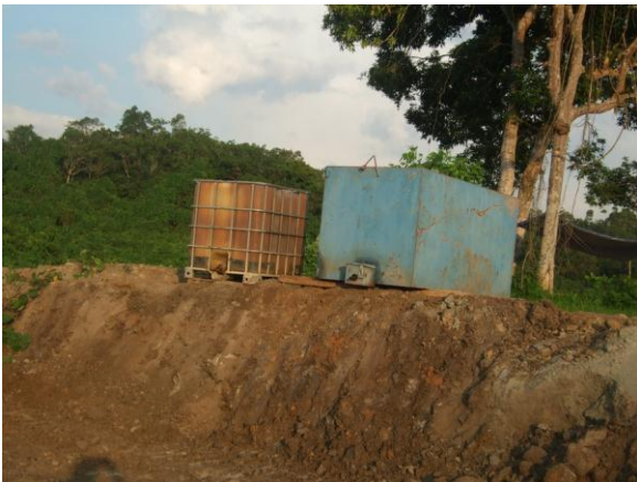
Site Fuel Storage
