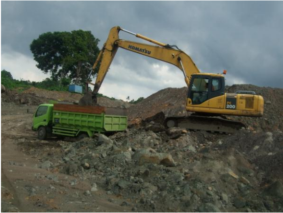
Pit extension – overburden removal
