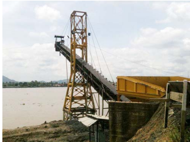
Image 2 – Transport Jetty used at Jongkang Project
