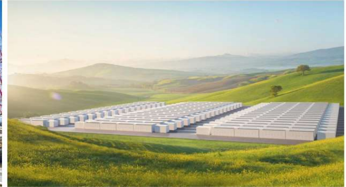
Moss Landing Energy Storage California
