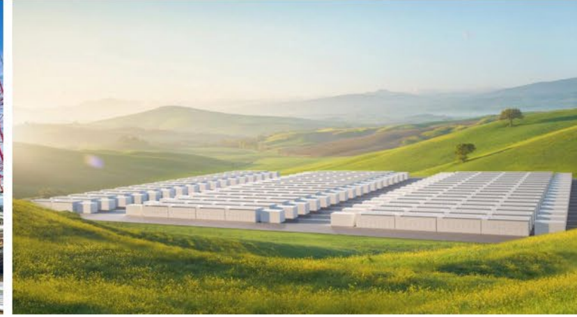
Moss Landing Energy Storage California
