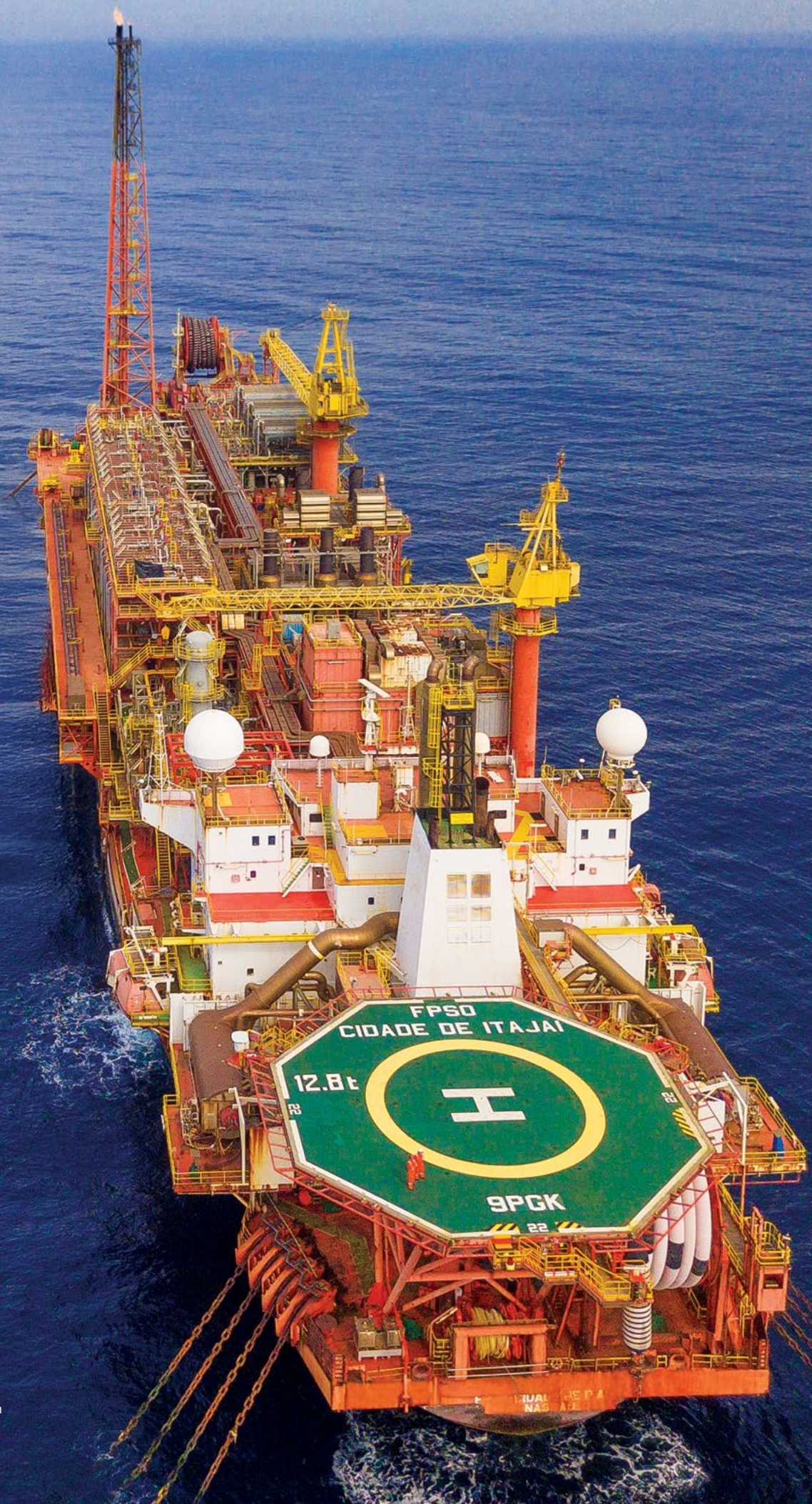
Baúna FPSO, Southern Santos Basin, Brazil
