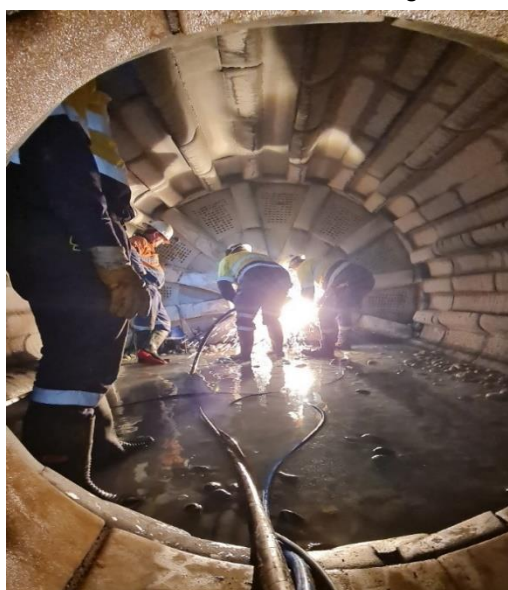
Figure 2 : Mill liner replacement works and visible gold embedded in liners prior to removal
