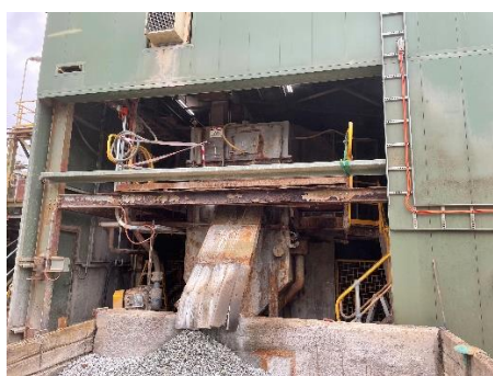
Figure 1. Old SAG discharge hopper
