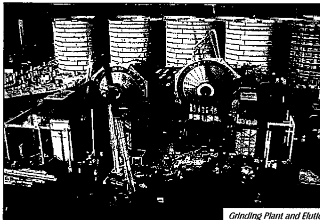
Grinding Plant and Elution Tanks under construction
