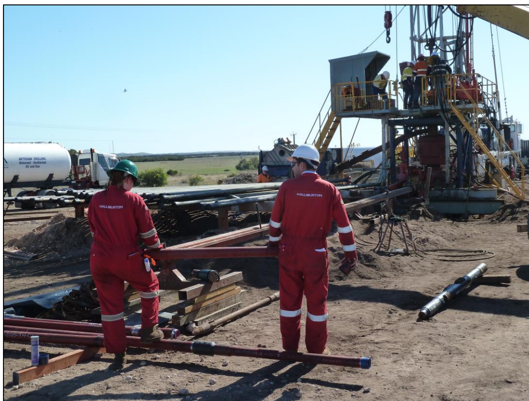
DCA, Key and Halliburton crew preparing to run production completion (above) and view looking north of rig floor (below) preparing to run in hole Westlog TCP guns and Halliburton completion equipment (foreground)
