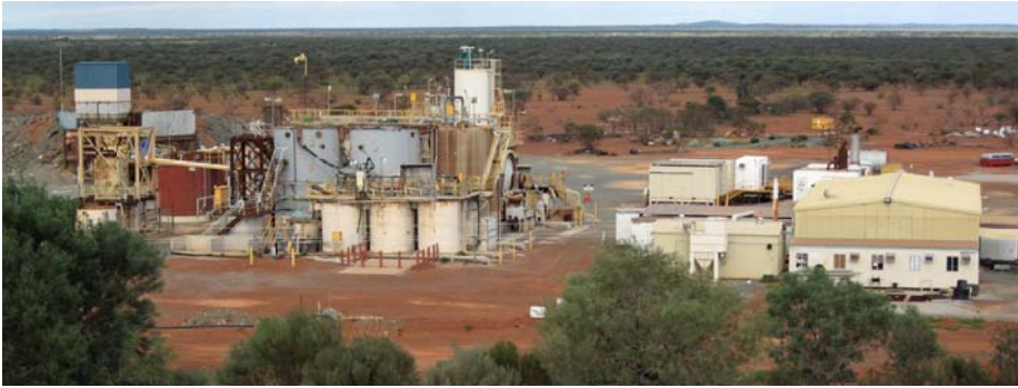
Figure 2 Burnakura CIL Plant
