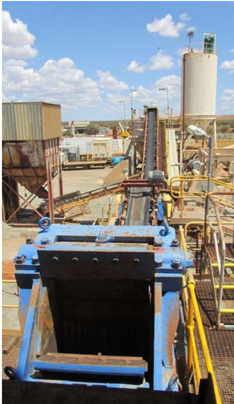
Figure 3 Primary crusher and ore conveyors
