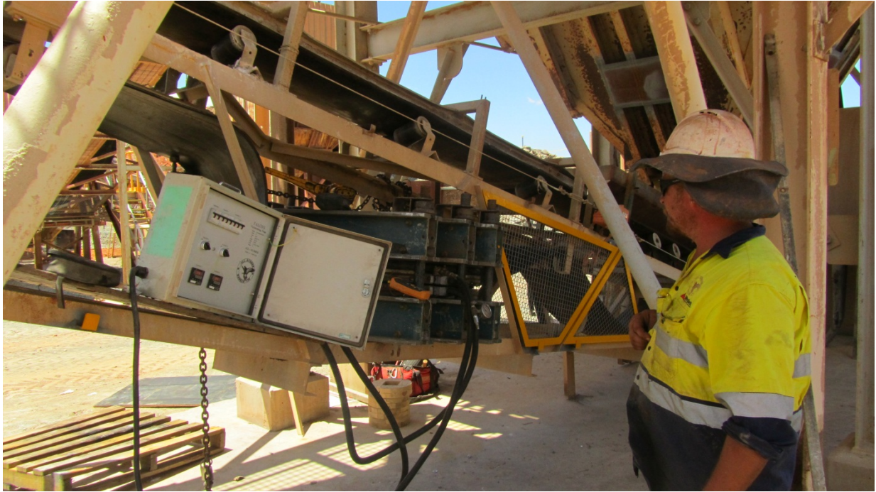
Figure 4 Installing new mill feed conveyor belting
