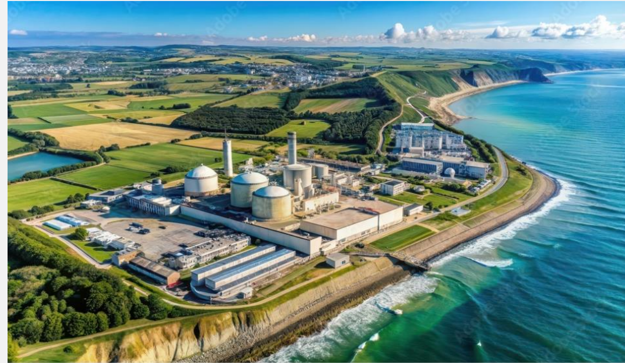
Nuclear reactor in Flamanville, France.
