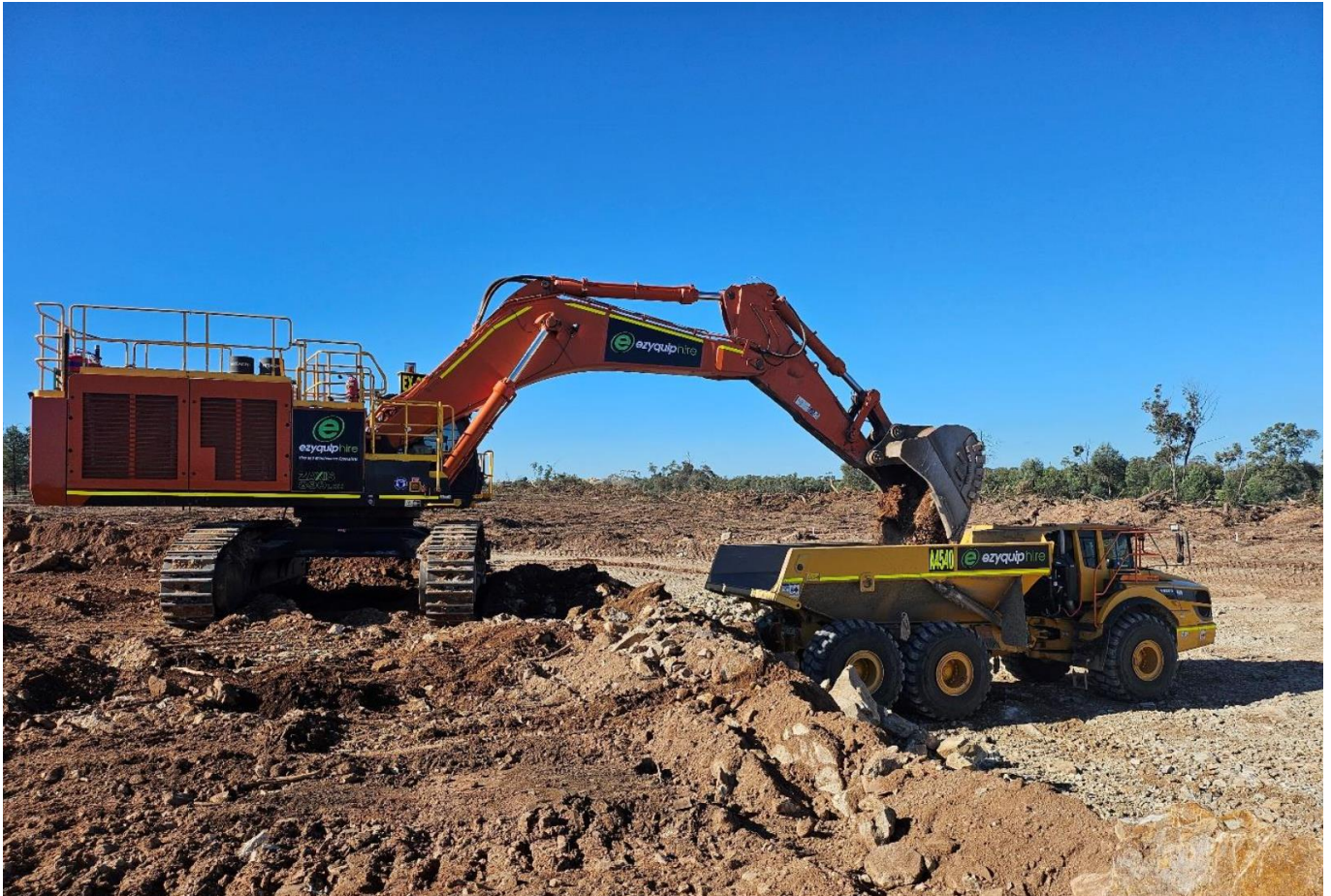
Figure 3: Open pit excavation and haulage.
