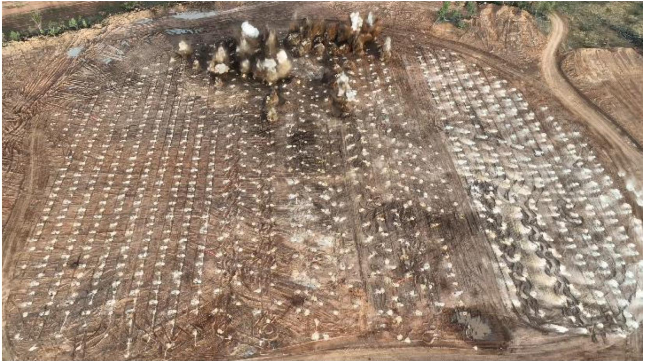
Figure 1: First blast at Pearse North open pit.
