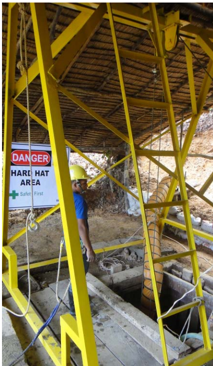
Temporary headframe and hoisting operation to support clean out and refurbishment of No.2 Shaft, Manuel Vein.
