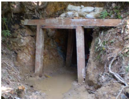
Exploration adit development.
