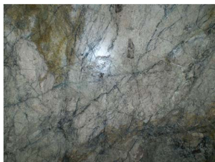
Covellite-bornite vein stockwork and disseminated style mineralisation. Adit 1, north face, Sabang Prospect (1.70% copper, 0.18g/t gold and 5g/t silver).
