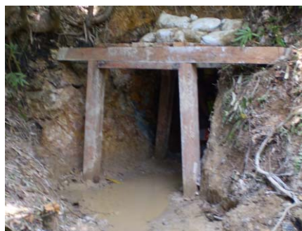
Exploration adit development.
